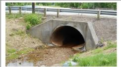
it is one of those pipes that allows water to run under a road. If this didn't exist, the water would pool and at times flood the road above. So with that image, let's read the quote.
